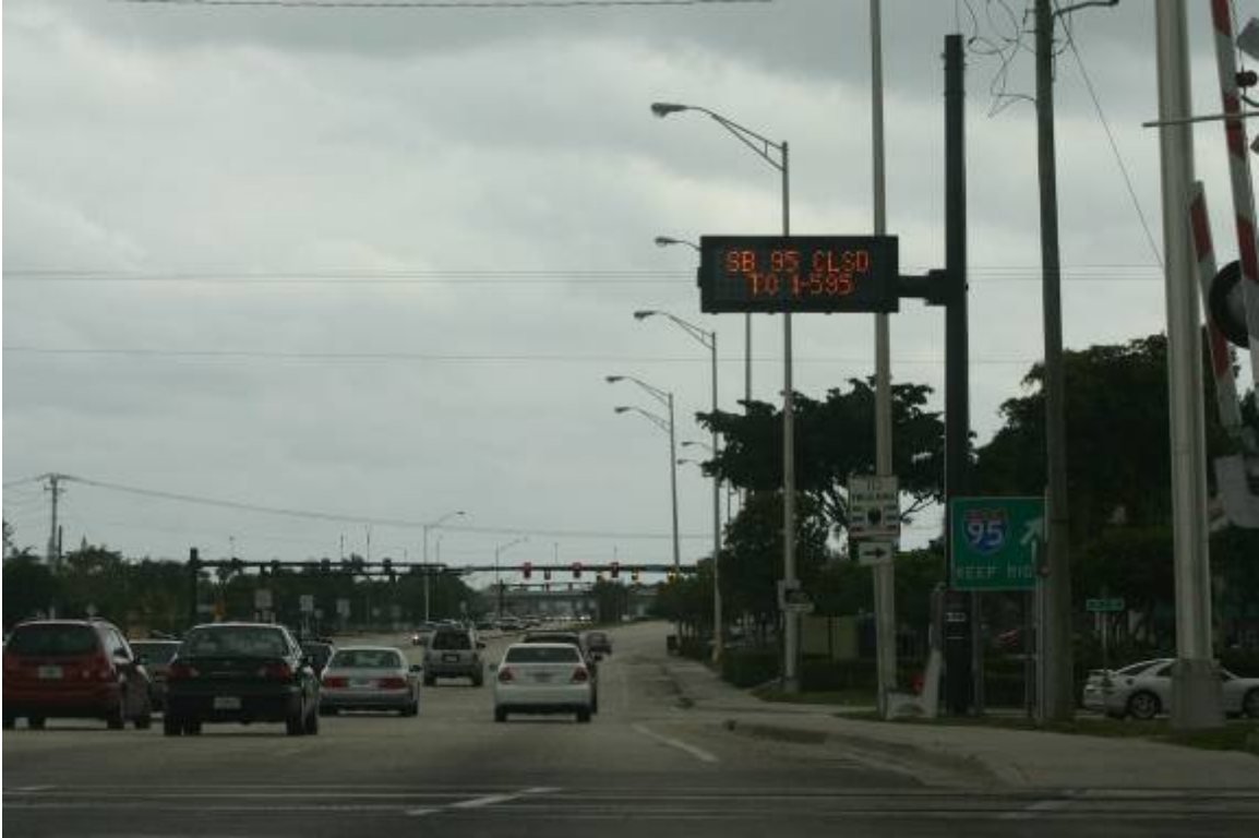
New arterial dynamic message signs will warn motorists of traffic conditions before entering the highway.
