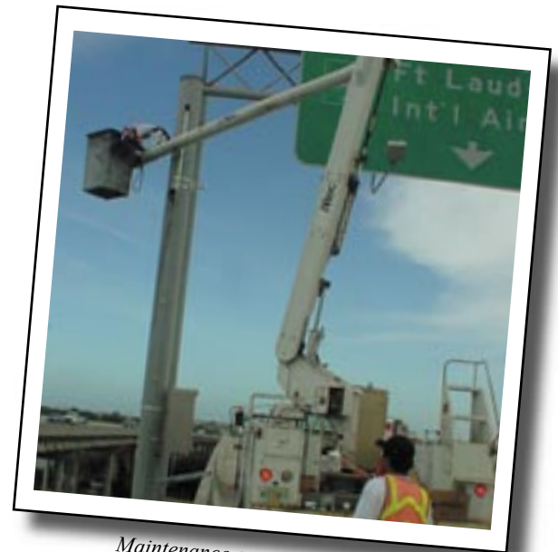
Maintenance contractors at work
