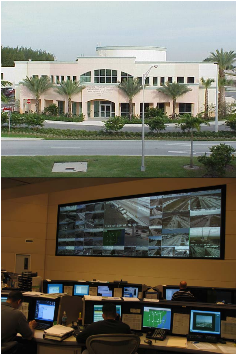
Figure 5 FDOT District Six SunGuide Transportation Management Center
